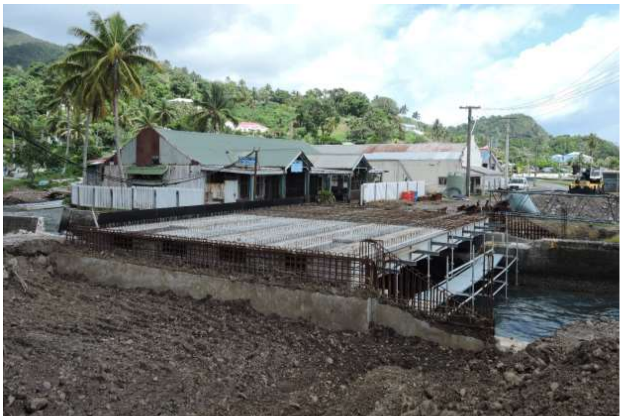
Picture Caption: works in progress at the Levuka Market Bridge
