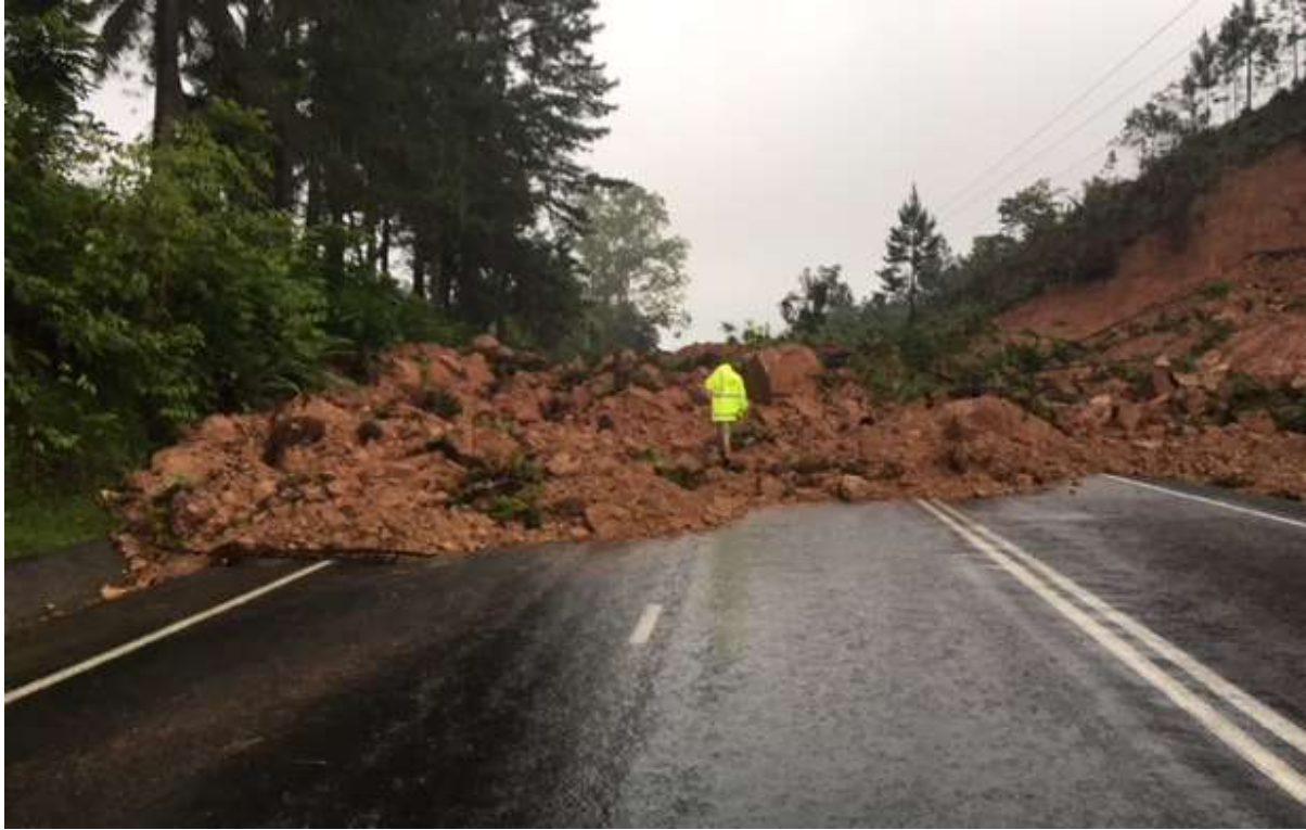
Photo Caption: Queens Road is closed at Veisari, Lami following a landslide early this morning.
