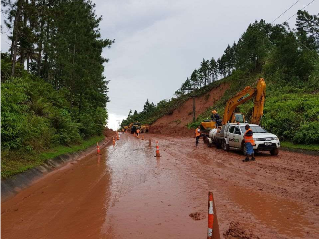
Photo Caption: Both lanes on Queens Road at Veisari, Lami is now open to traffic.
