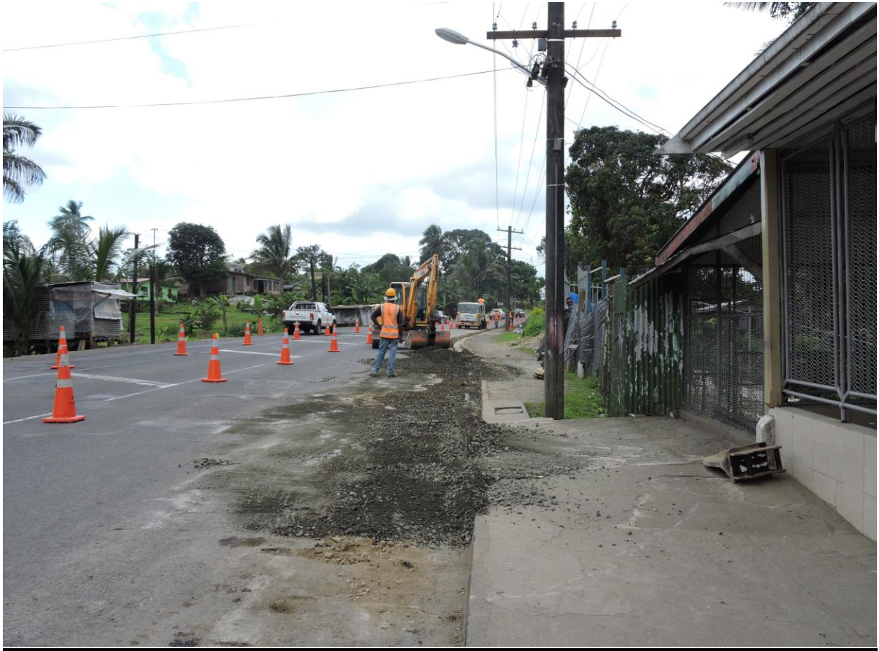
Picture Caption: FRA is carrying out major pavement repair works at Princes Road (from Lakeba Street to past Khalsa Road junction).
