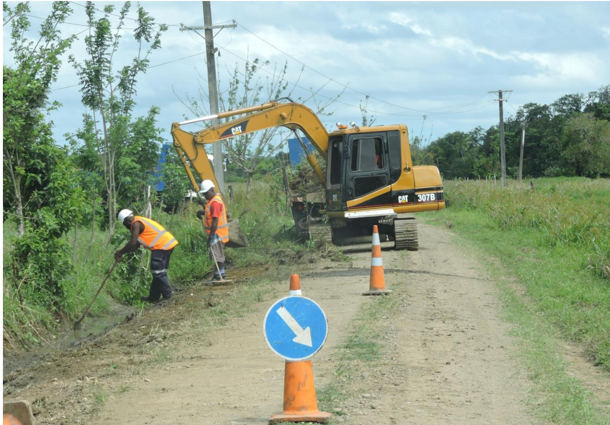
Picture Caption: FRA contractors clearing the roadside drains and overgrown vegetation on the road reserve at Nabilo Road in Korovou.
