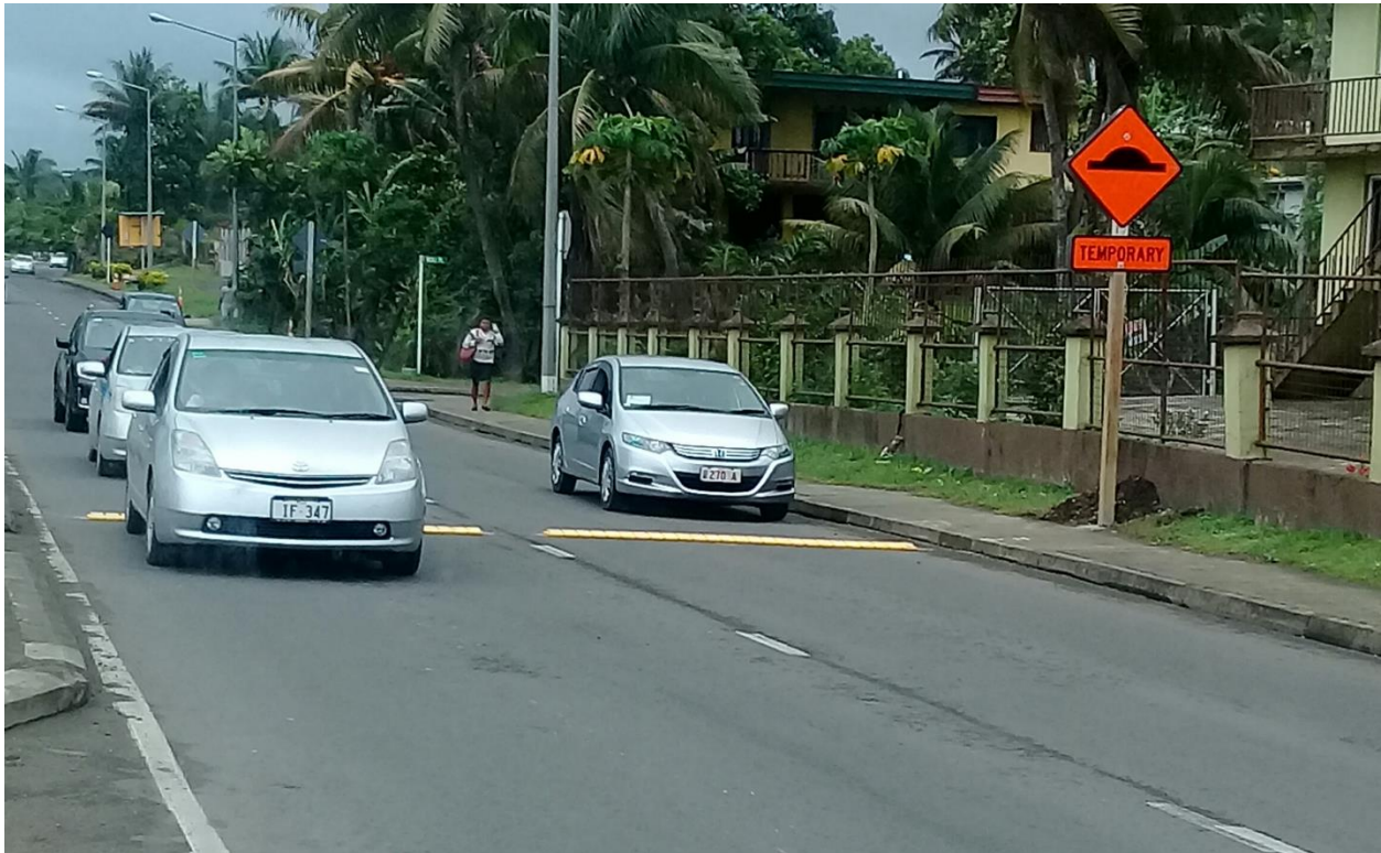
Picture Caption: FRA installs temporary road humps in front of Vivras Plaza, Laucala Beach Estate to address speeding concerns.
