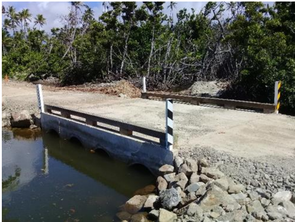
Photo Caption: The new and improved culvert crossing in Vanuabalavu
