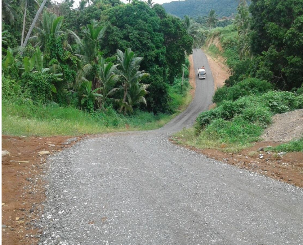
Picture Caption: The successful completion of the new road in Moala
