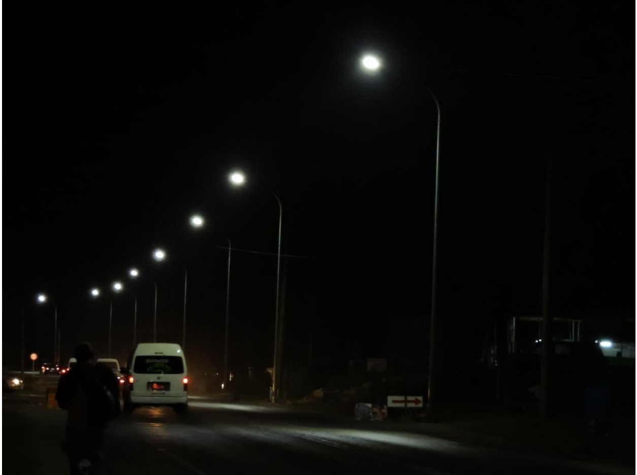
Photo Caption: The newly installed streetlights in the Western Division
