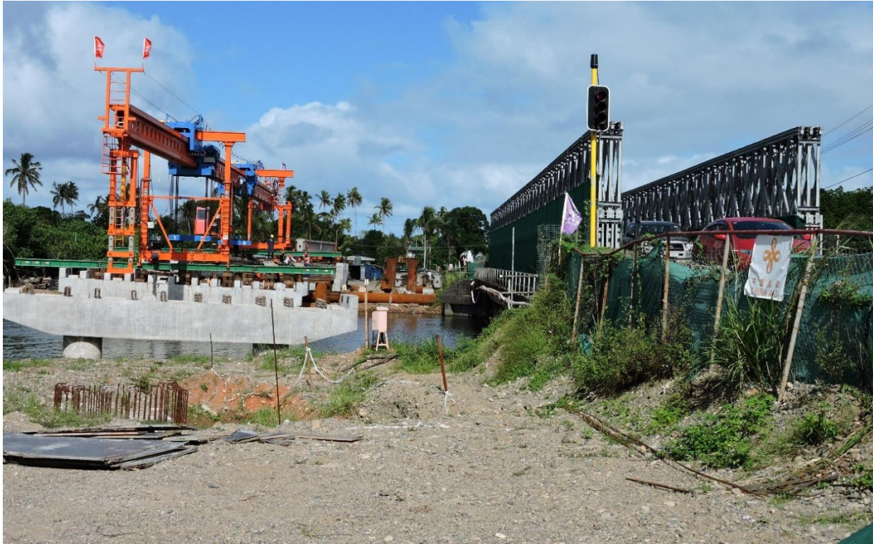
Photo Caption: Construction of the new bridge alongside the existing bailey bridge.
