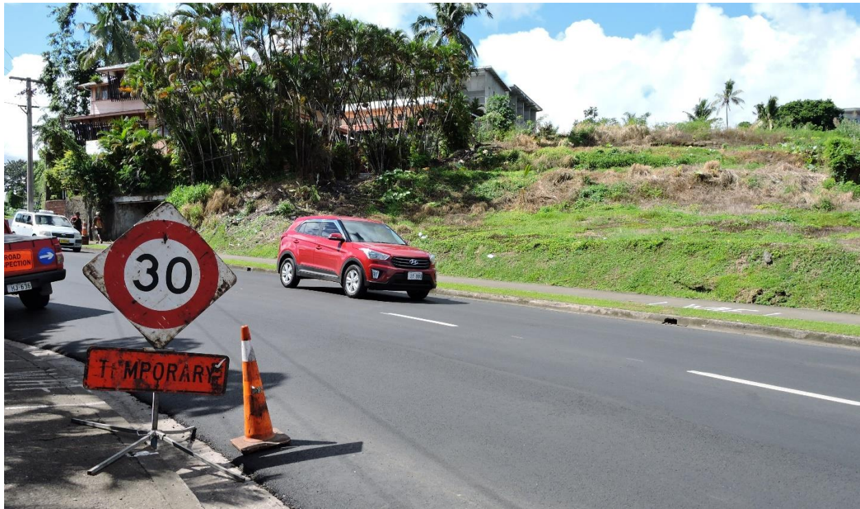
Photo Caption: Road surface improvement work at Waimanu Road in Suva
