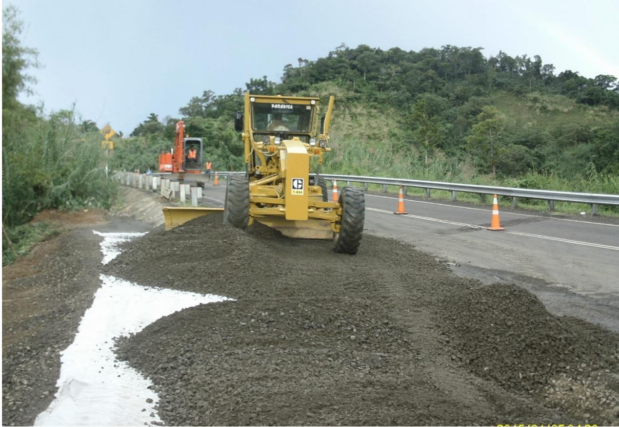
Clearing the road side carriageway for the diversion route.
