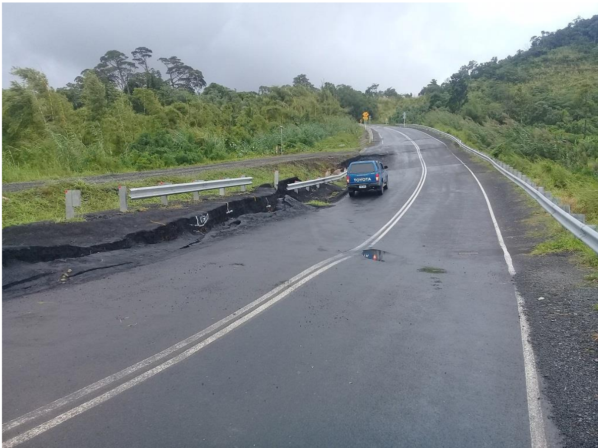
Further movement has been recorded on the Lomaloma Stretch
