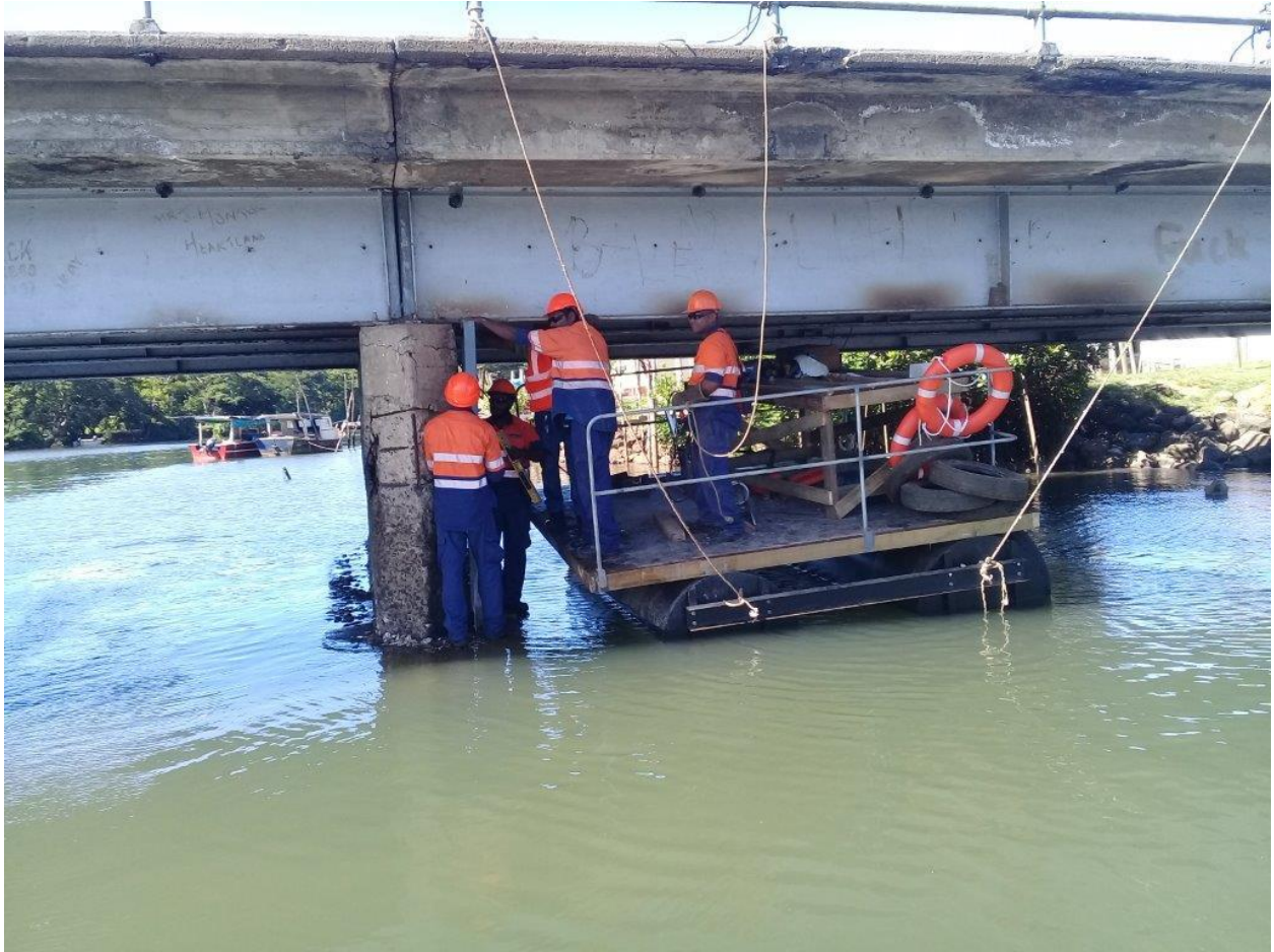
Photo Caption: Labasa Bridge will be undergoing urgent repair works from tomorrow (May 1 st ).
