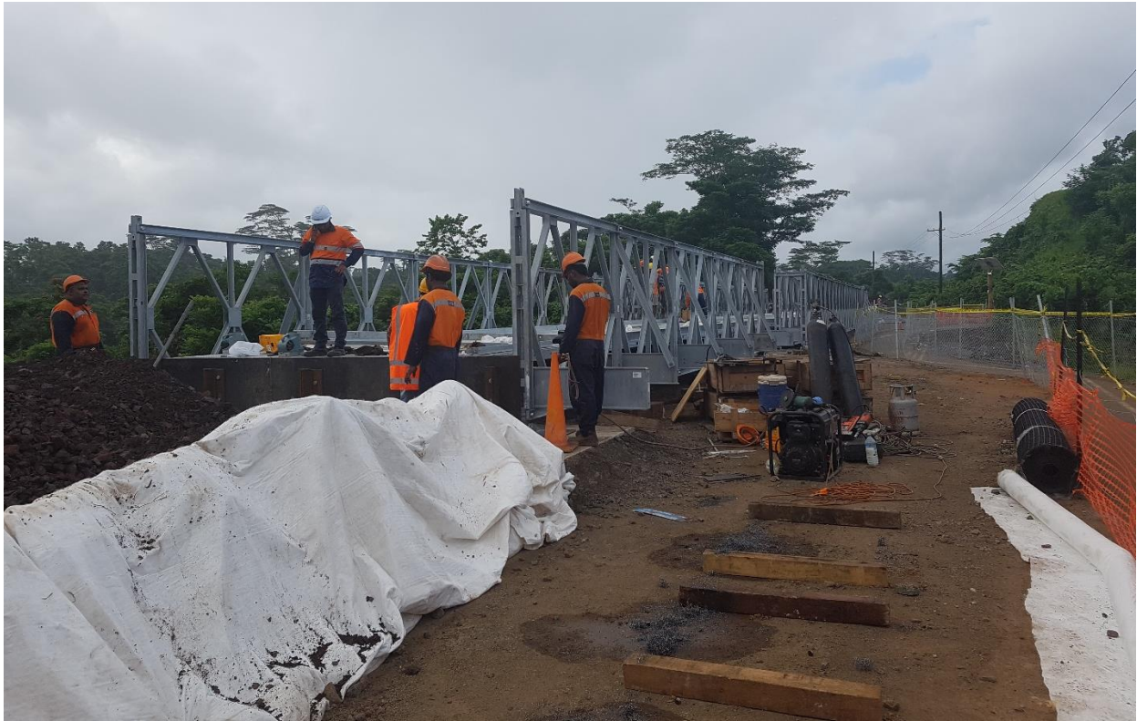
Photo Caption: Installation of Bailey Bridge in Kasavu, Tailevu in progress.
