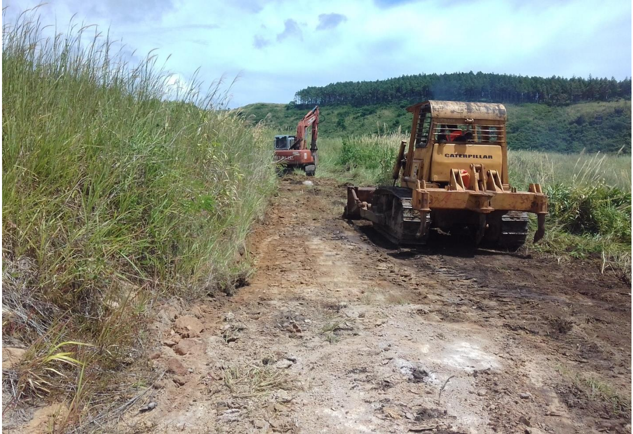
Photo Caption: Works have commenced at Yawe Road in Kadavu
