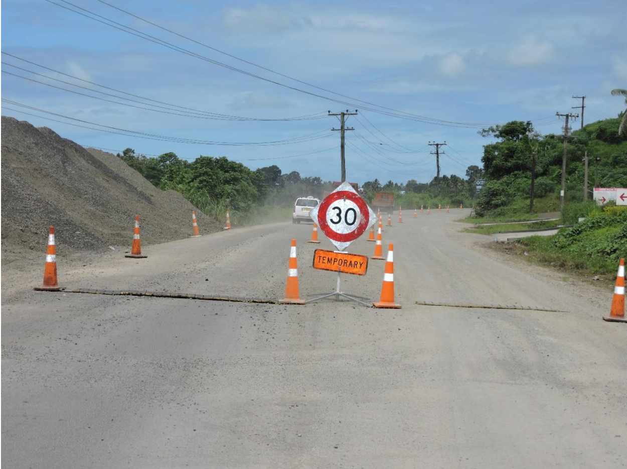
Image 4 – Motorists advisory sign, temporary 30km through active construction site.
