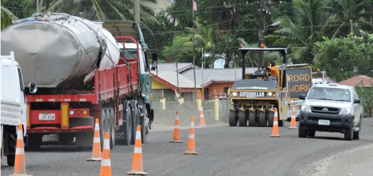
Image 3 – Road works taking place at Waila on Princes Road.
