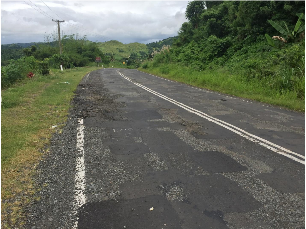
Photo Caption: Extensive sealed road failure near the Naiserelagi Village in Ra.
