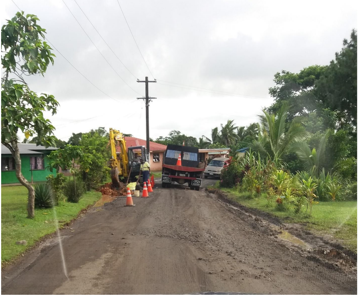
Photo Caption: Water works carried out this week at Mara Road through Raralevu Village.
