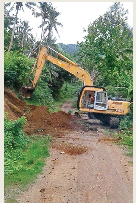
Heavy equipment was shipped to Gau to clear the roads.
