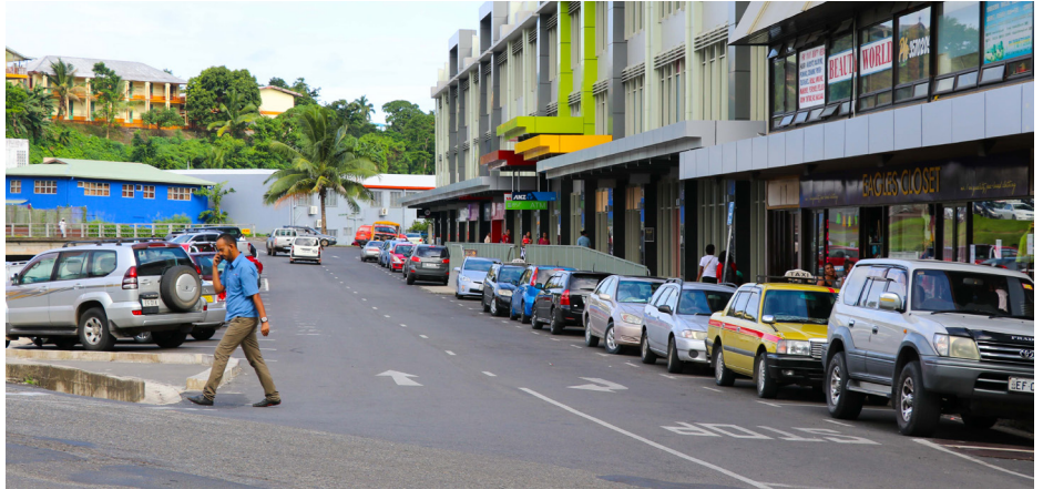
The Greig Street renewal work has upgraded vehicle and pedestrian access.
