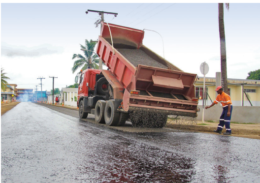
Sealing Rawasa Road.
