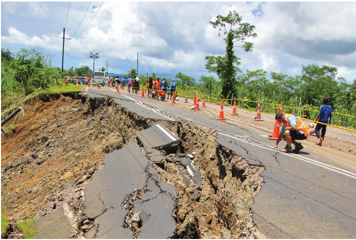
The slip at Kasavu on Kings Road.
