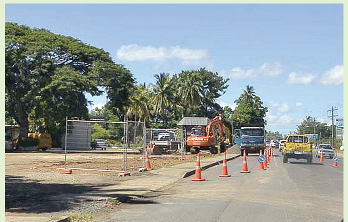
The four-lane project underway at Martintar.
