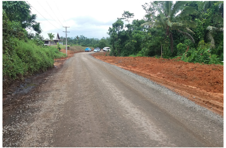
The Bau Tikina detour has been opened, keeping communities accessible.
