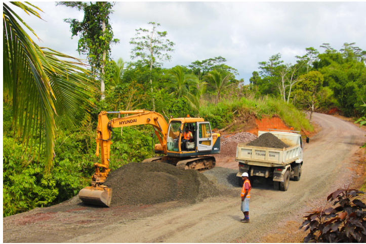
FRA contractors working to open the Bau Tikina detour.
