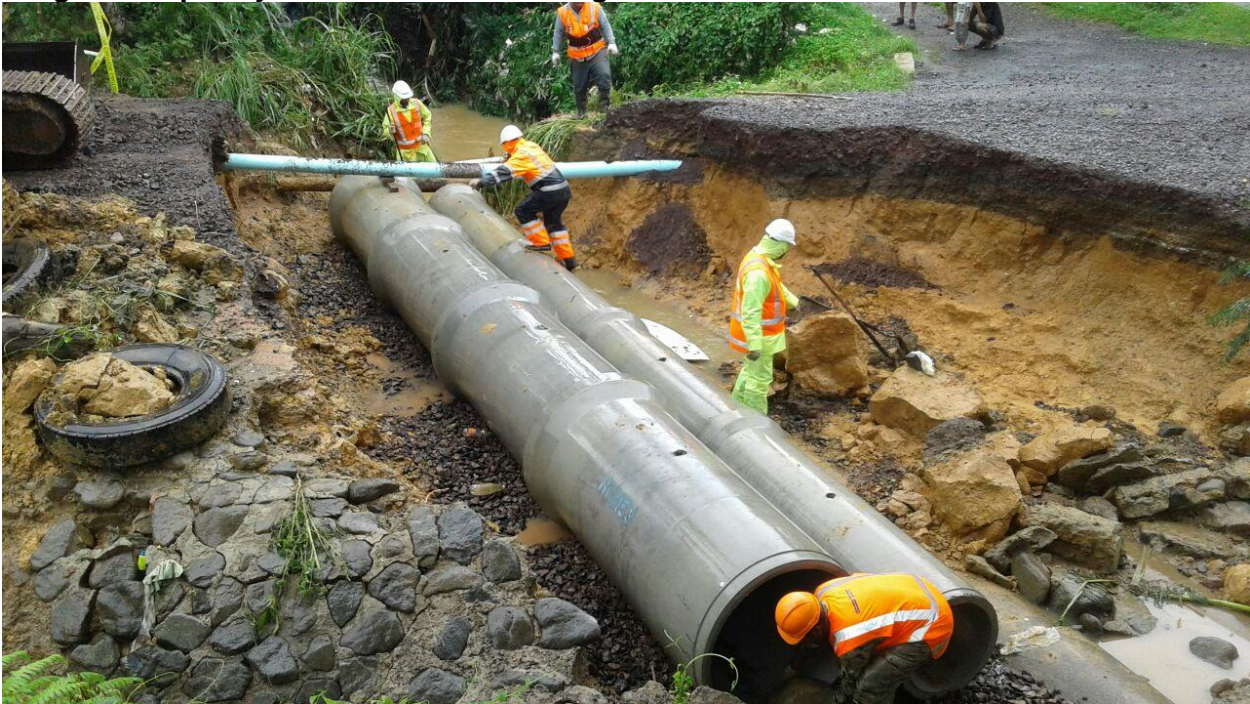
Image 3 Temporary reinstatement work begins on 17 th December 2016
