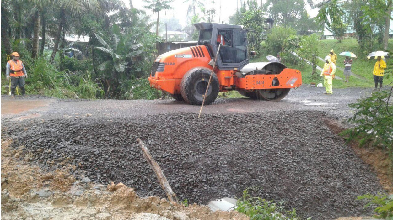
Image 4 Temporary reinstatement work begins on 17 th December 2016
