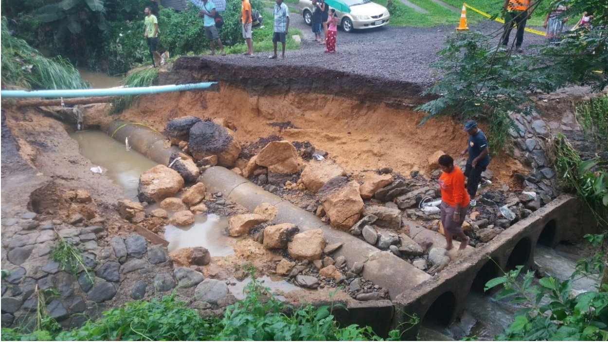
Image 2: Culvert washout during TD04 in December 2016
