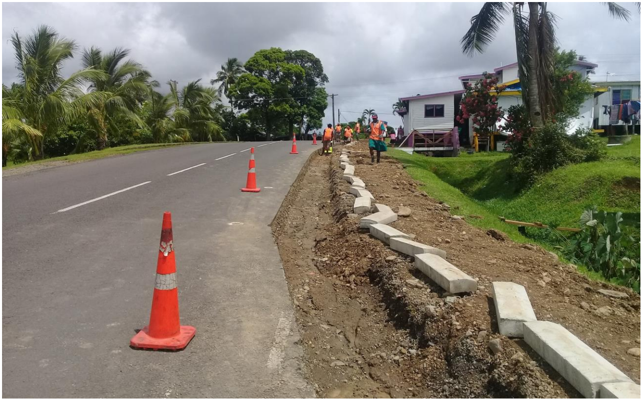
Photo Caption: Construction of new footpaths in Cunningham.
