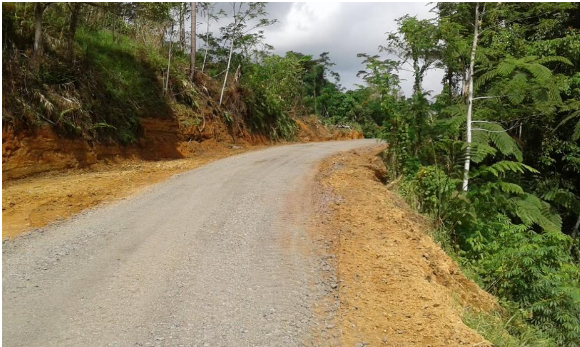
Photo Caption: Work in progress at Bau Tikina Road off Kings Road.
