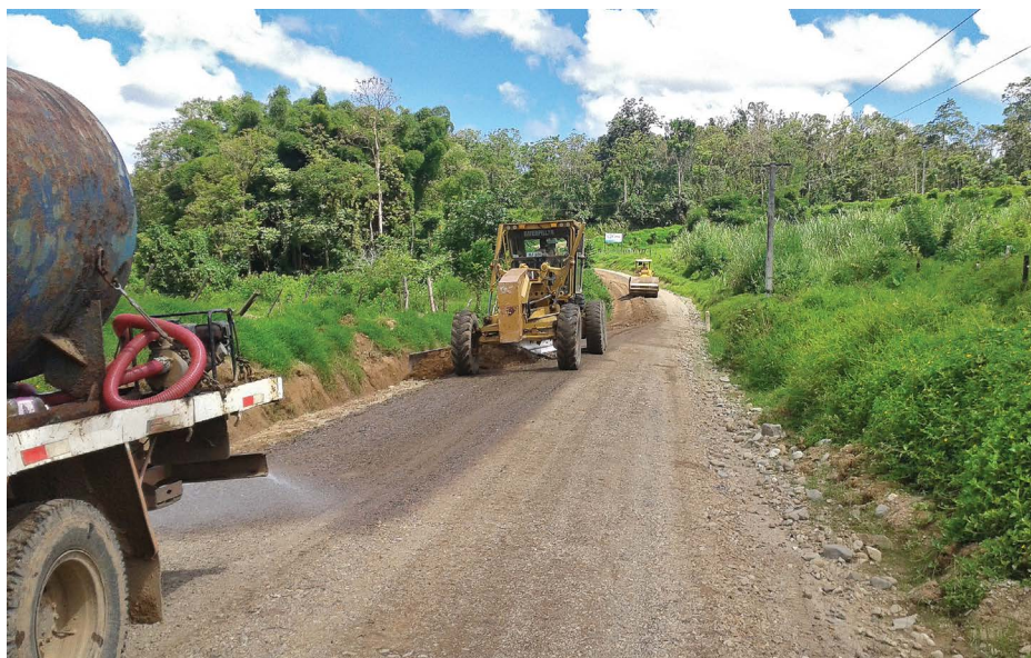
HSHSL carries out resheeting work in the Central Division.
