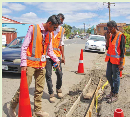
FRA Cadet Engineer, Mr Kunal Nand (left), inspects work in Lami with Hot Spring Hire Services staff members.
