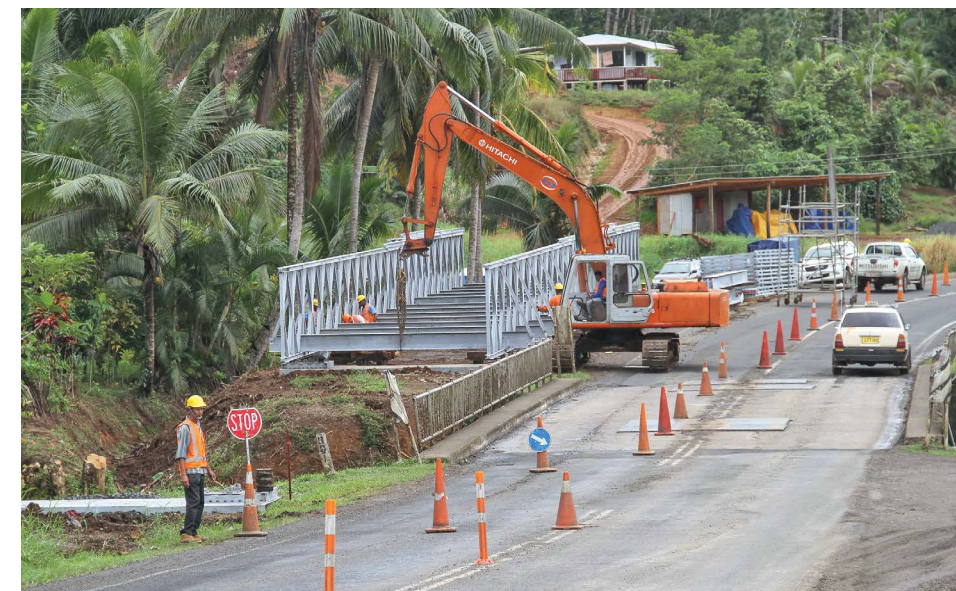
Installing the Bailey Bridge alongside the Vugalei Bridge on Kings Road.
