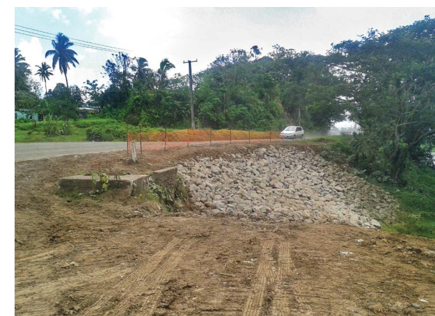
Slip repair on Kadavu Island.
