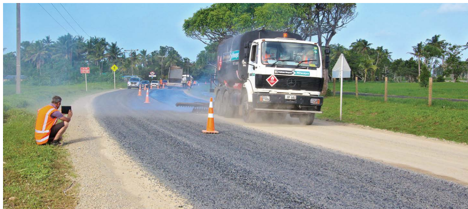
Resealing Queens Road at Pacific Harbour.
