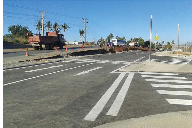
A recently opened section of the Namaka corridor.
