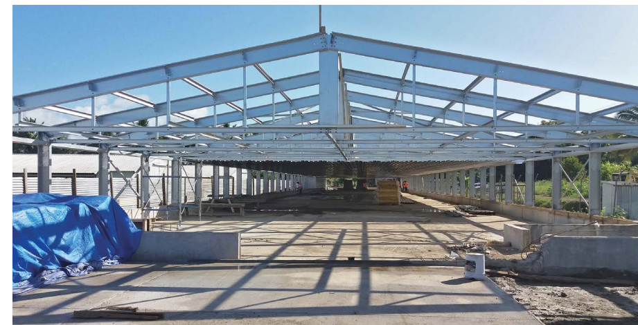
HSHSL at work on construction for the Goodman Fielder company.
