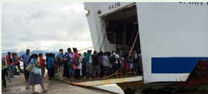
The new, safe Natovi jetty will benefit hundreds of passengers using it daily.
