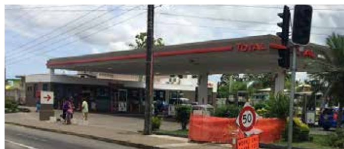
Careless driving damaged the traffic light control box at Makoi causing weeks-long inconvenience.
