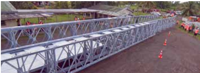
Bailey bridges will be used as temporary and emergency response structures.
