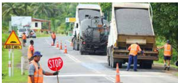
Rehabilitation prolongs the design life of a road.
