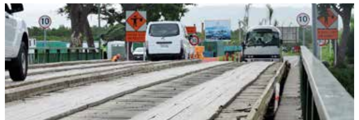
Pacific Marine and Civil Solutions has started work on Denarau bridge.
