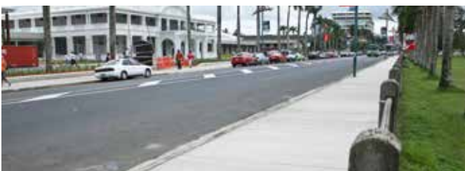
New standards will guide all road-related upgrade and construction works.
