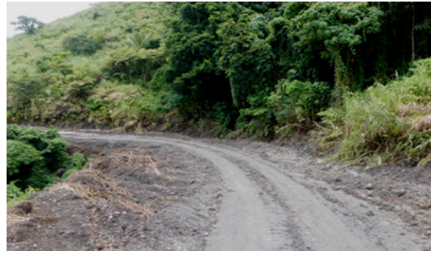
These before and after photographs of Baidamudamu Road on Kadavu show how overgrown some roads have become, and the difference that grading and resheeting makes.
