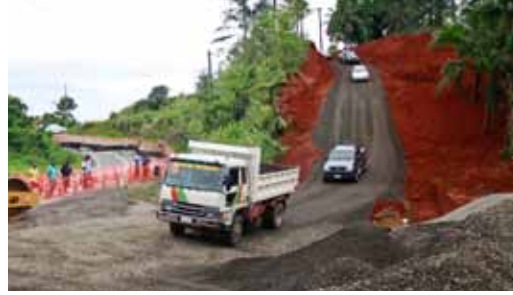
Single lane, steep access on an alternate route opened within 24 hours of the slip
