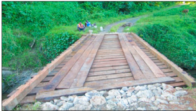
Bucalevu bridge, Taveuni, after it received urgent repair.
