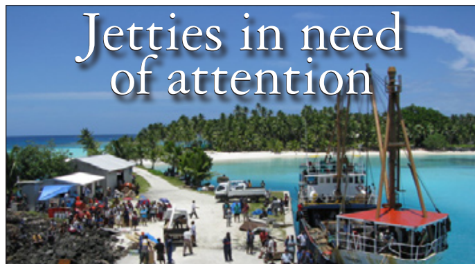
Rotuma Jetty provides a vital link in connecting the island with the rest of the world.
