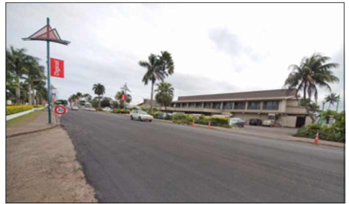
The FBM process has contributed to rapid construction in the Suva CBD as seen here outside the Holiday Inn.
