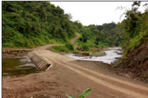
Thurston Road was included in the Suva CBD Rehabilitation programme. A new Irish crossing to Namosi Village was constructed after the old crossing was destroyed by Cyclone Evan.
