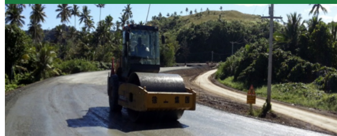
The road is compacted to maximum density while keeping the centre highest so water will drain away.
