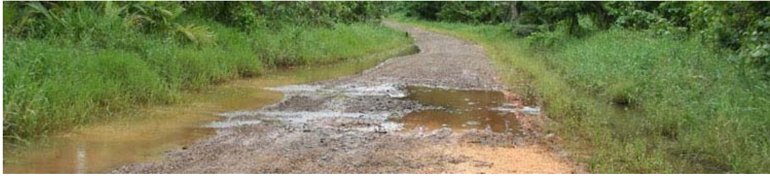
Figure 10: Example of road deterioration due to poor drain maintenance, Savusavu
